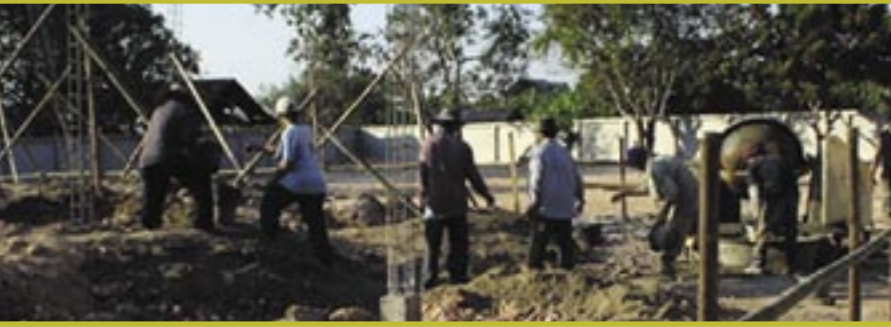
Foundations are put in place
